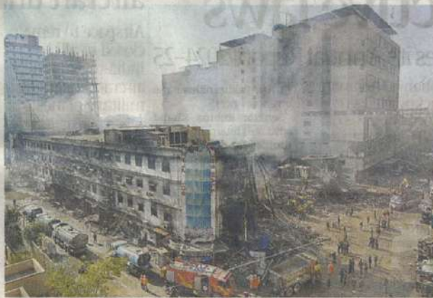
LIFE AMIDST RUBBLES: Rescue workers search amid the debris using excavators after a massive fire at a shopping mall in Karachi. PHOTO: AFP
